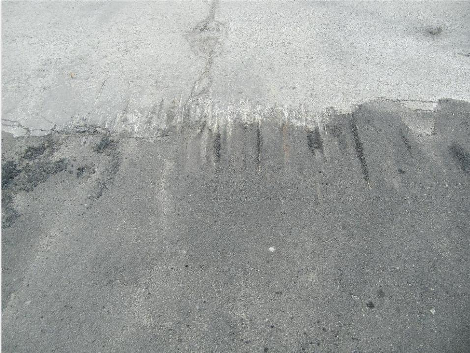
View of multiple scrapes on south edge of depression on Vancouver Street in London, Ontario on April 25, 2014. Road construction was temporarily filled to cause the depression likely leading to many incidents of damage to the vehicles of drivers passing over the depression.
